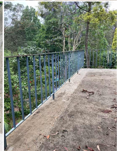
Concrete spalling and erosion to metal balustrade.
