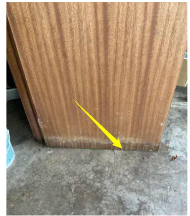
Minor water damage to garage storage door.
