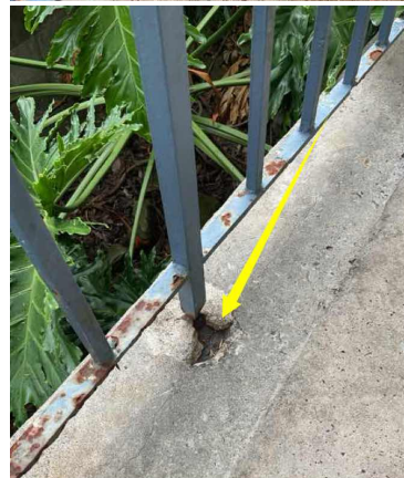
Concrete spalling and erosion to metal balustrade.
