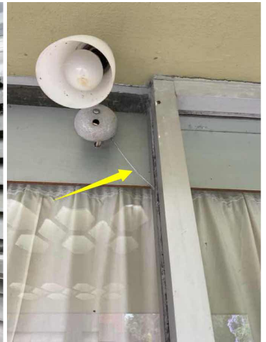
Glazing putty has deteriorated.
