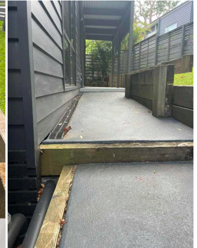
Concrete path falling towards the home.
