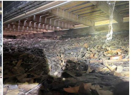
Timber decay evident. Underside of decking.
