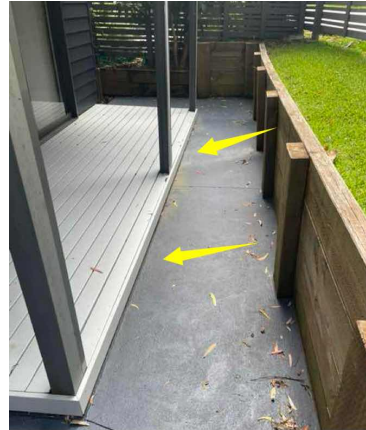
Concrete path falling towards the home.
