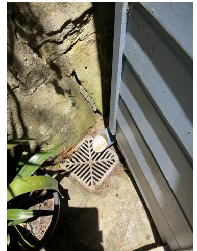
Not the best practice to channel stormwater beneath the property in this manner.
