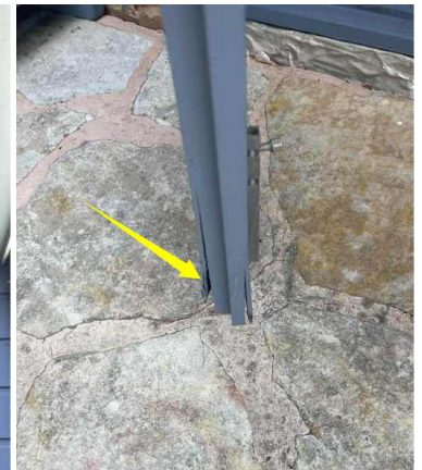
Water damage to cellar access door.
